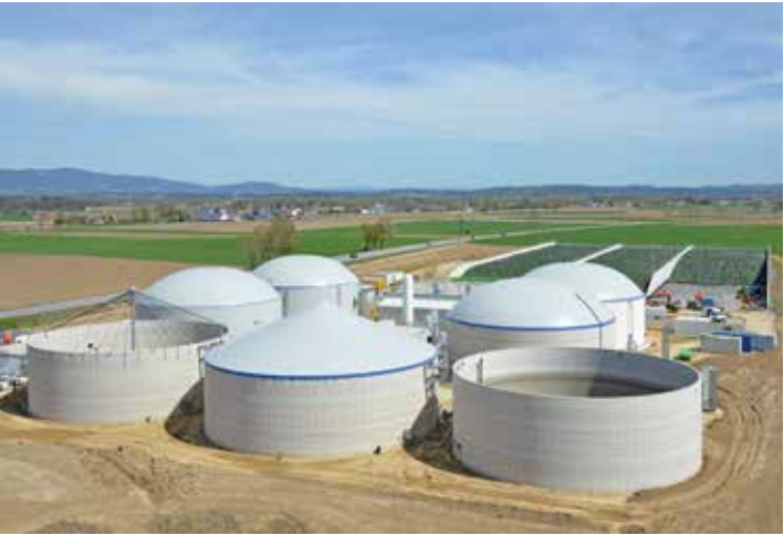
Biogas facility – slurry management and energy recovery for sustainable farms
