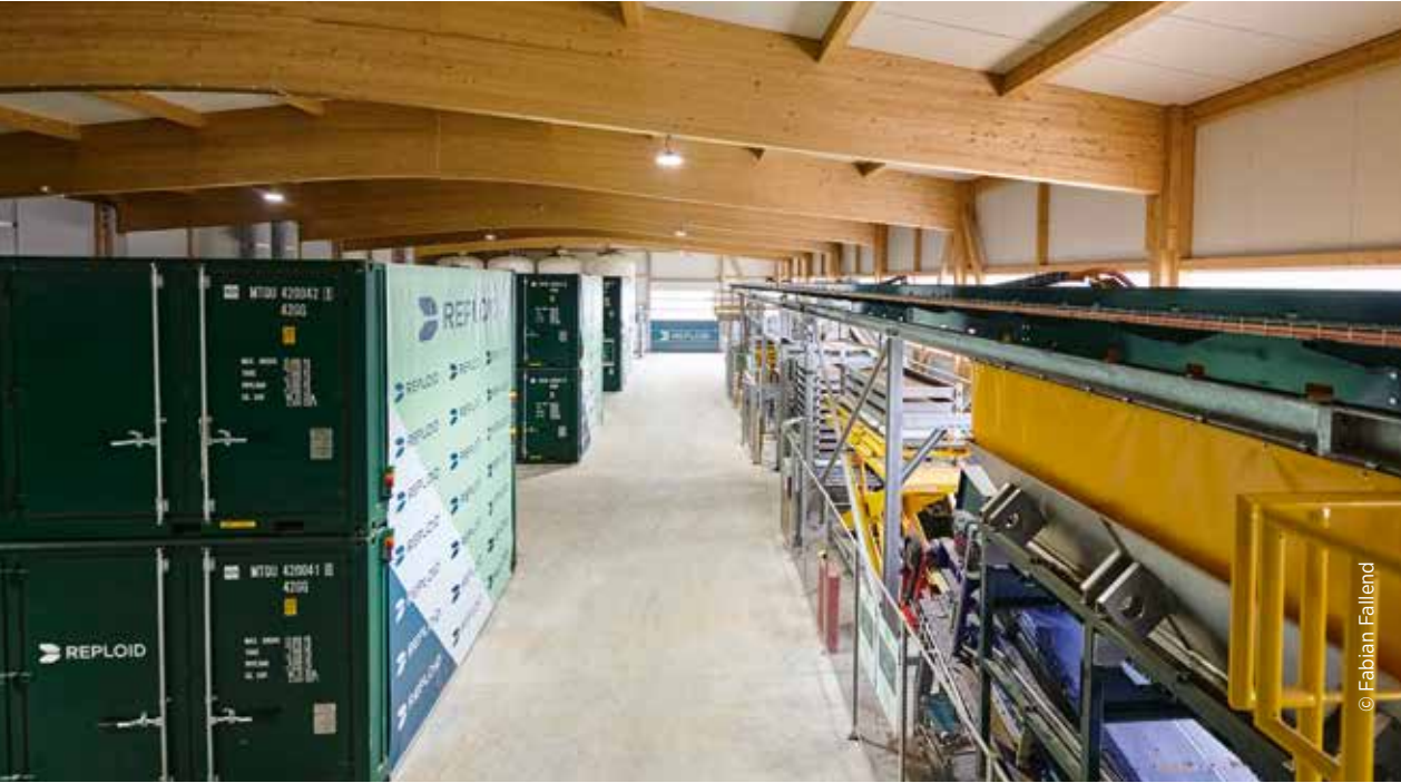
From waste to value: a highly-automated ReFarmUnit on a compact 24 x 60 meter footprint
